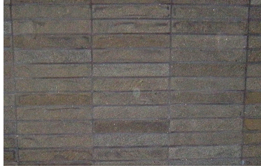
Finger Split Stack Bond Cut
